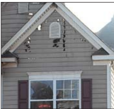
A fireman walks through a second-story window in the Bennett home.
