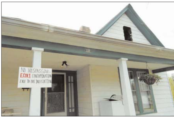
DANGEROUS SITUATION: A sign warns visitors of the dangers of E. coli coming from years of bat guano that have been piling up in the ceiling and walls of the house.
